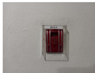
Fire Alarm Manual Station
